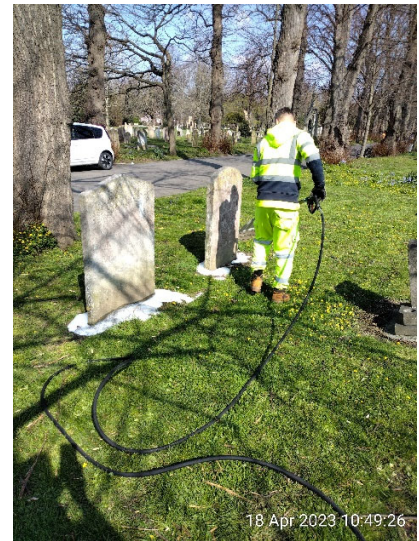
Treatment around headstone bases to reduce strimming.
