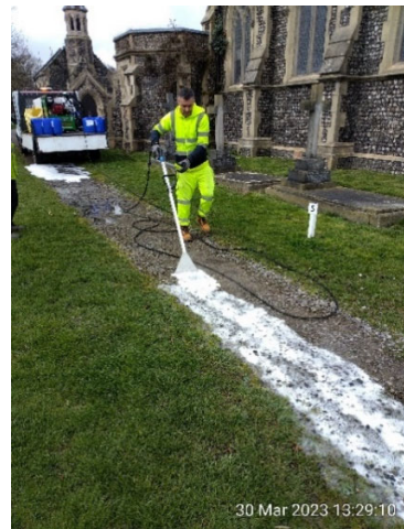
Operative showing trip hazard of hose and residual foam 10 mins after operation.
