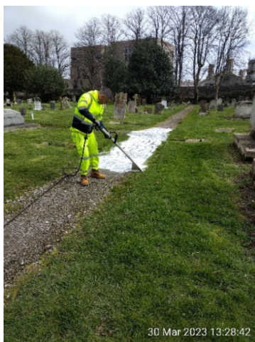
Operative showing trip hazard of hose and residual foam 10 mins after operation.
